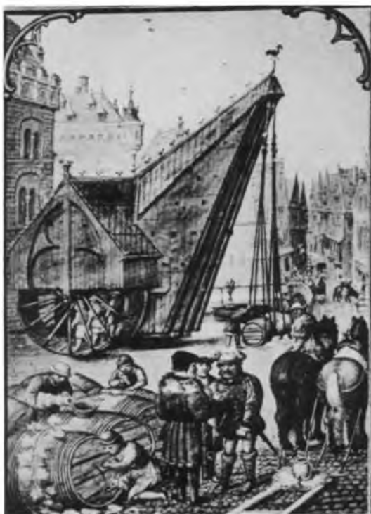
28. Hoist operated by tread-wheel, 16th c. (p. 168 n. 125)
