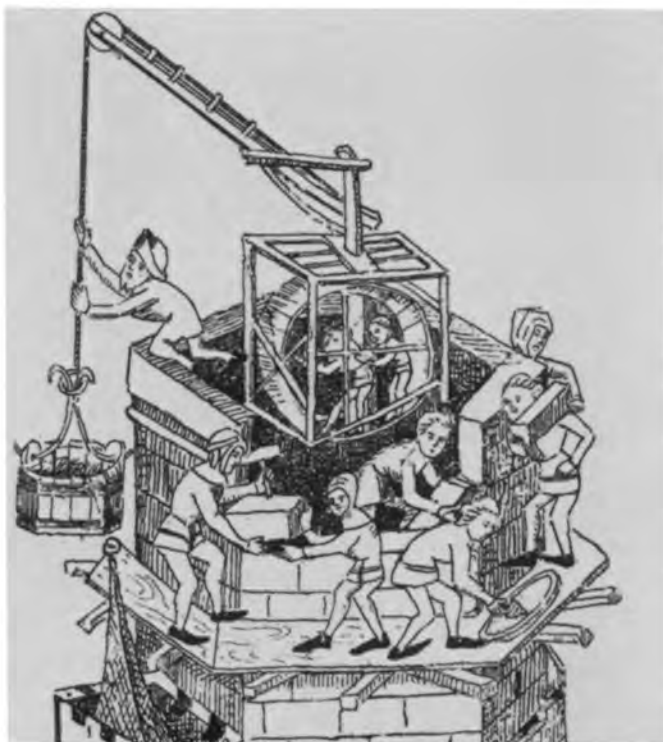
27. Hoist operated by tread-wheel, 14th c. (p. 168 n. 124)
